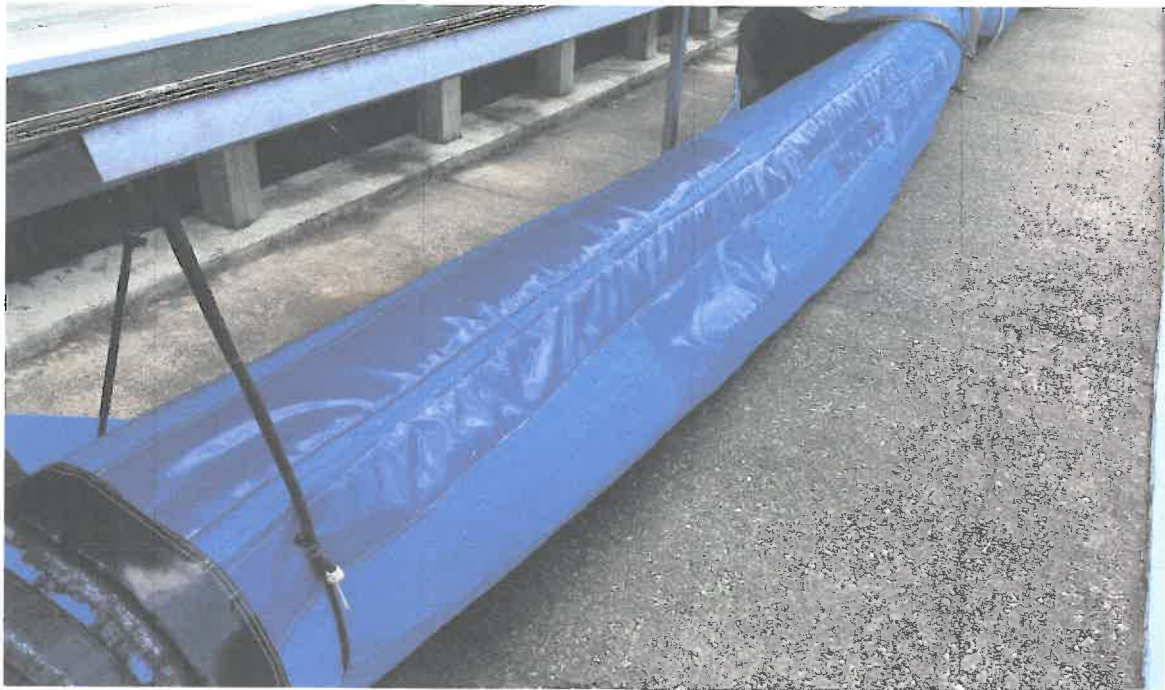
One of the covers that has been temporarily repaired
